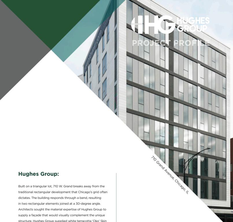
structure. Hughes Group supplied white terracotta 'Oko' Skin by Rieder to wrap the sides of the building and the shifted openings. The two ends, one of which is the street front, are contrasted by glass window walls with varied metal finishes.
